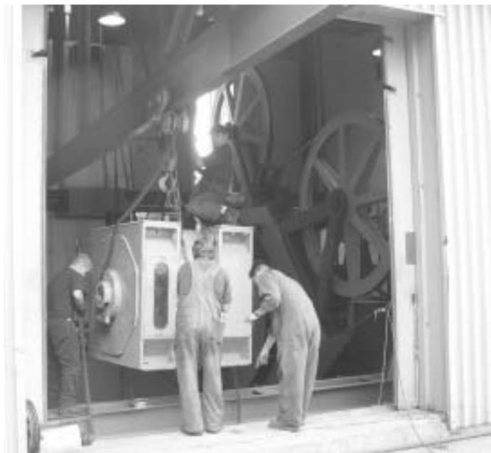
During the scheduled Tramway maintenance that ended Monday, workers received the system's 900-horsepower motor after refurbishment work at General Electric, then winched it into the building through a back door at the Tram station, and into place to pull the haul cables.
