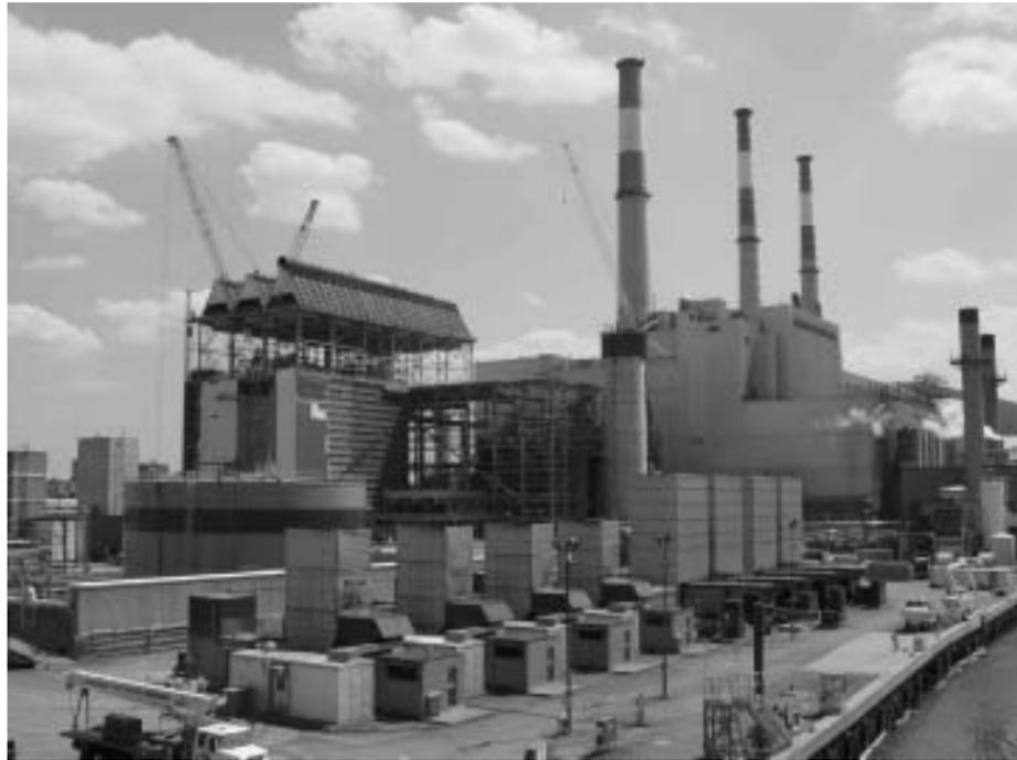
Keyspan concluded that 400 feet was "sufficient to allow the plume to escape the downwind, turbulent 'cavity' zone caused by the air-cooled condenser." The cavity height was determined to be 322.5 feet, she said, "and therefore, the proposed stack height is sufficient to keep the plume out of the cavity."
